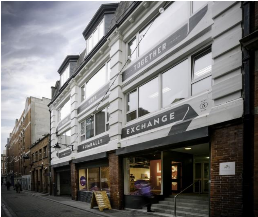
Photo of Structure
